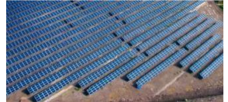
Ground Mounted Solar
