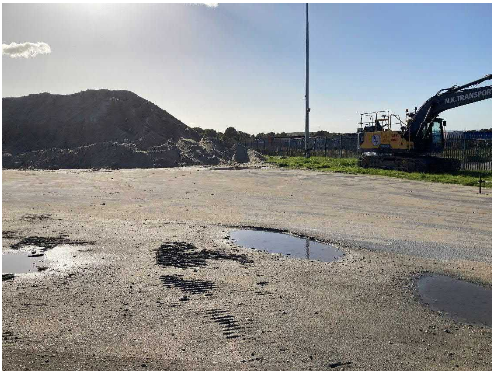
Photograph 4. Hard standing and rock salt storage pile in northern Survey Area.
