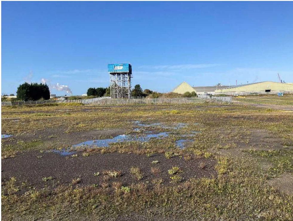
Photograph 3. Bare ground/ ephemeral vegetation in southern Survey Area (with water tower in background).
