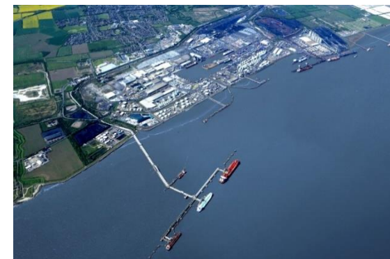
Viking: CCS shipping and pipeline terminal
